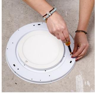
Shut off the main electrical supply at the fuse Screw the metal base to ceiling using installed box/circuit breaker.
