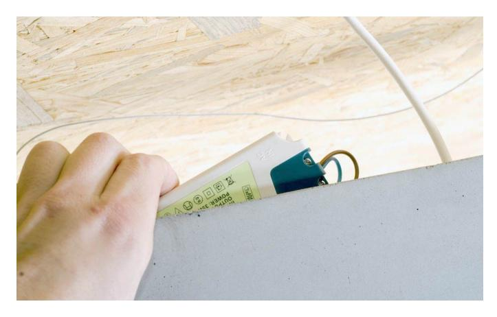
6. Elevate the ceiling rose part and move it as close to the ceiling as possible.
