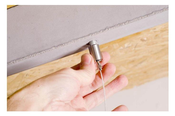
7. Screw the metal parts with the stoppers to secure the part position.
