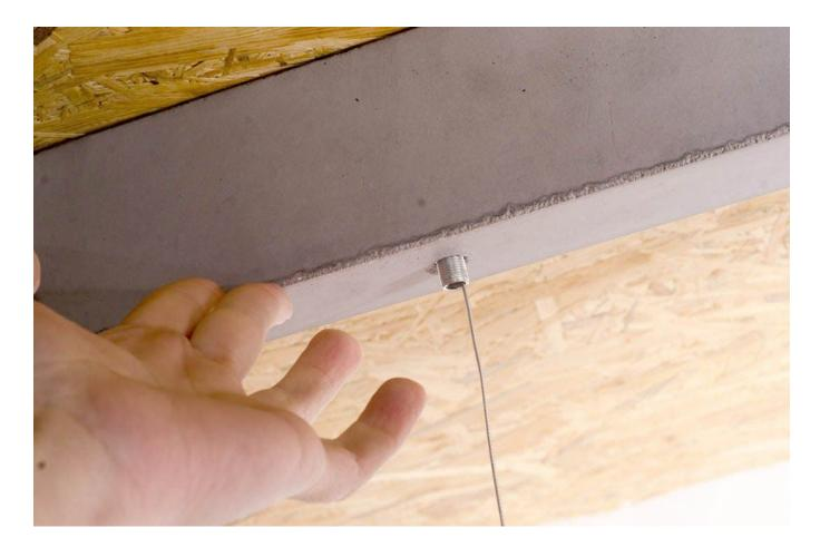
5. Lift the ceiling rose and hide the driver inside with the wires.
