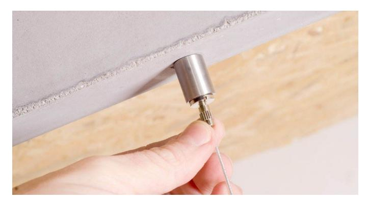
8. Level the lamp with the stoppers. Push it towards the ceiling to make the line loose. Secure the position by screwing the stopper safety cap.
