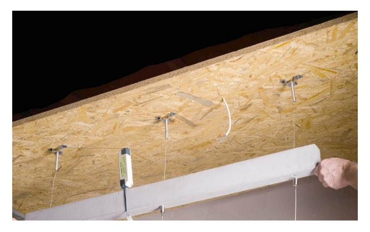
3. Mount the elements to ceiling then twist in the long, threaded sleeves. Be sure to lift the lamp during the process.
